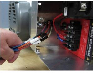
3a. Mount Enclosure (Idler/floor) & Idler Wires: Remove idler conduit cover and pull the idler wires through the enclosures rear hole after installing the snap bushing.
