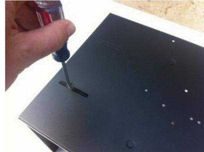
Locate the 4 slotted knockouts on the bottom of the control panel enclosure. Be sure to completely remove the remnant strip. If remnant strip drops into enclosure, maneuver enclosure until remnant strip can be removed.
