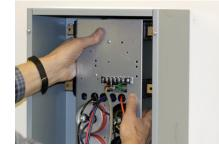
After cleaning out the enclosure, reinstall the controls using the 4 lock nuts provided.
