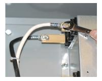
Using the Bolts and Lock Nuts provided, secure the ring lugged wires to the proper bus bars. Torque the bolts to 25 in-lbs.
