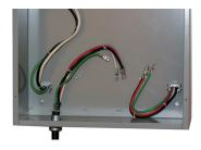
Pull electrical lines into the enclosure. Run the ground lines with each circuit. Make sure to leave enough wire to reach the bus bars.
