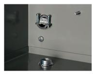
Mount enclosure on secure wall or machine. Attach conduit fittings for 1-phase input line, 3phase line to idler and 3phase line to load.
