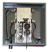
A complete installation should be neat and clean with plenty of wiring space.
