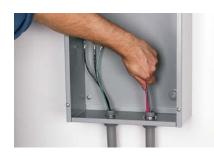
**3.** Pull wires through conduit. Leave enough wire for connecting to busbars. Terminate wires with a ring lug that takes a 1/4 inch bolt.
