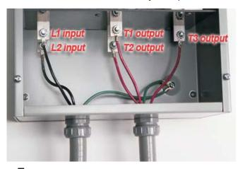
**5.** Bolt the wire terminals to the busbars using the 1/4 inch bolts and nuts provided. Ground the enclosure. If terminals come closer than ½ inch to each other, insulate them.
