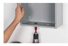
**2.** Mount enclosure to wall or other suitable structure with (4) 1/4 inch fasteners.
